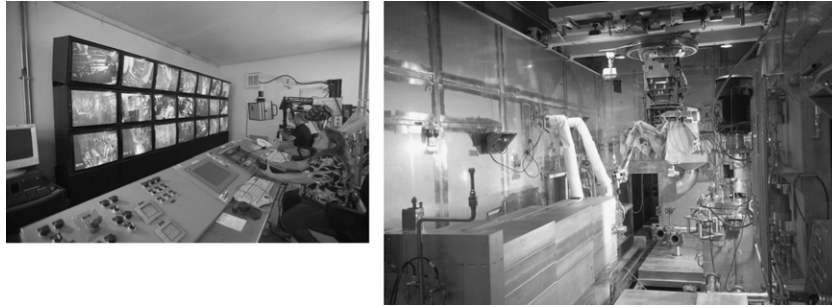
Fig. 12. Remote handling control room and target service bay.
