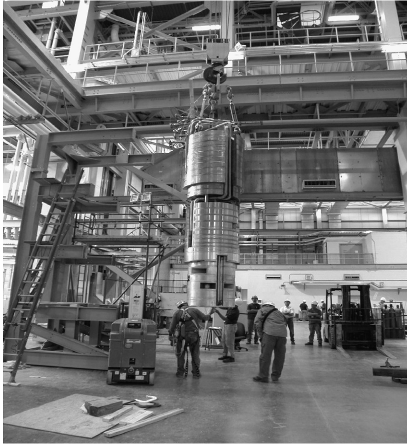
Fig. 8. IRP lift for installation after repairs.
